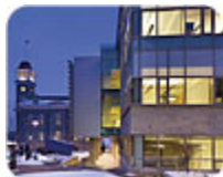
Cambridge City Hall, Photo by Tom Arban.
