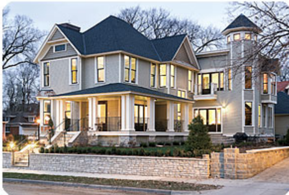
Colfax Ave. S. Renovation, Photo by Troy Thies Photography.
